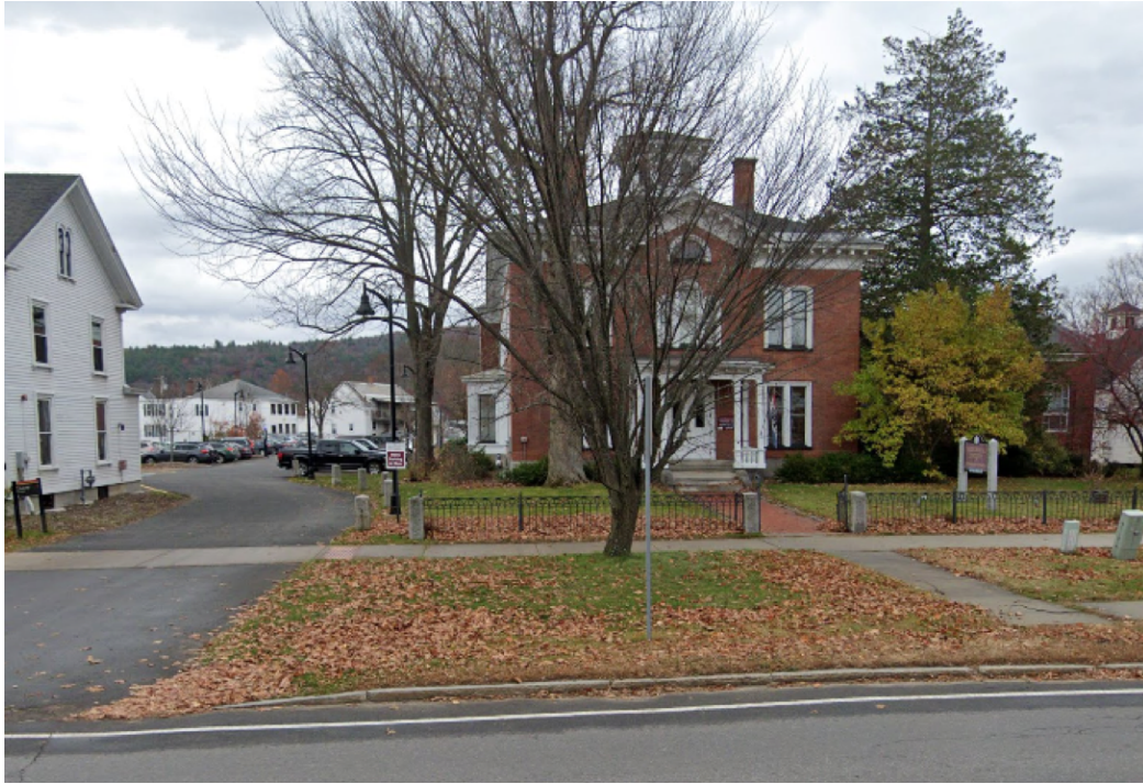
Figure 1. View of Historical Society Building
